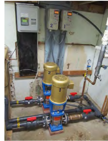
Well water system recently upgraded with new pumps that feature variable frequency drives
