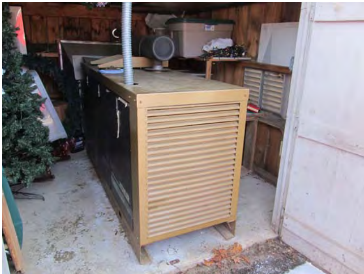
Propane-fired emergency generator serving community building and well water pumps
