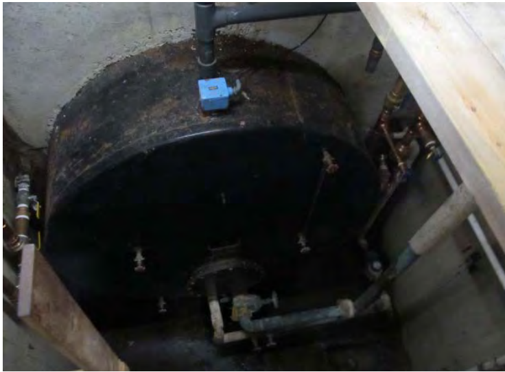
Nose section of original underground steel storage tank that serves the development's well water system
