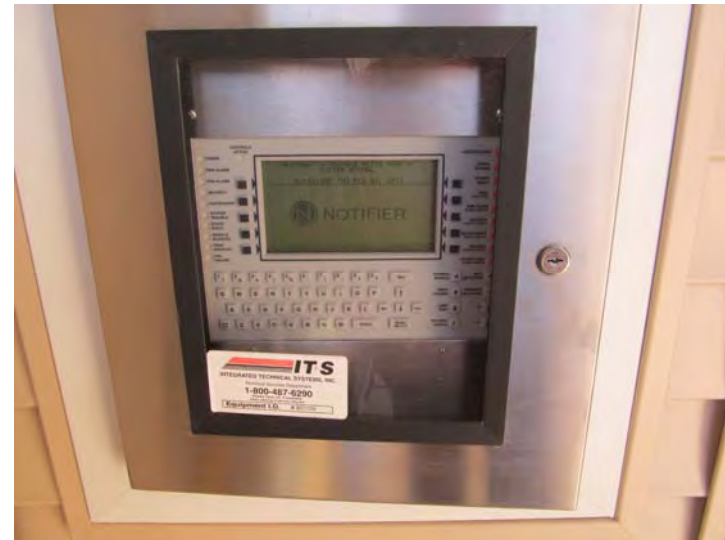
Recently upgraded fully addressable fire alarm control panel located at community building
