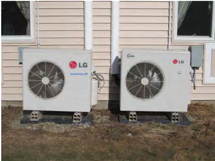
Typical exterior, air-cooled, condensers for heat pump systems recently installed in all units
