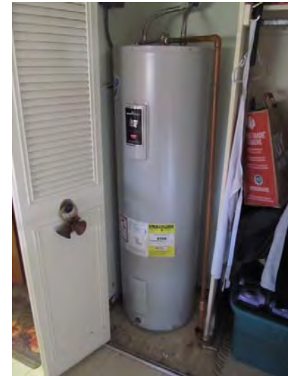
Typical unit-level electric domestic hot water tank
