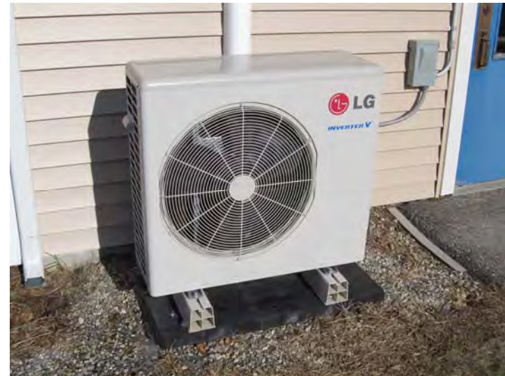
Typical exterior, air-cooled, condenser for recently installed heat pump systems serving community building
