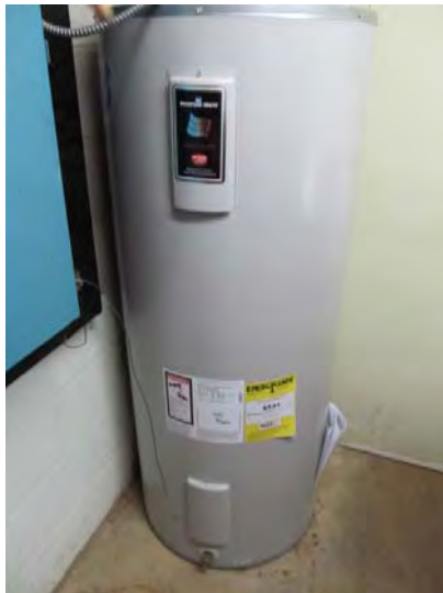
Electric, storage-type, domestic hot water tank serving common areas at community building
